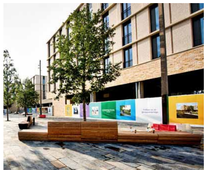
Figure 2: Successful temporary hoarding to retail at Eddington.
